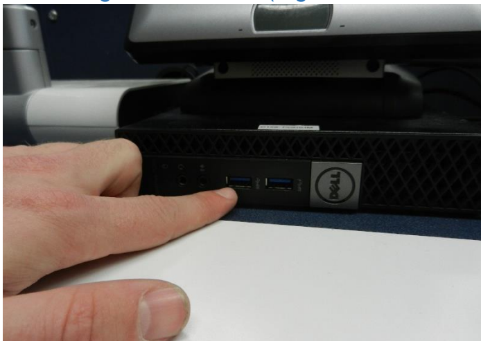
Figure 8: SVSU USB Ports Under Master Control Unit
